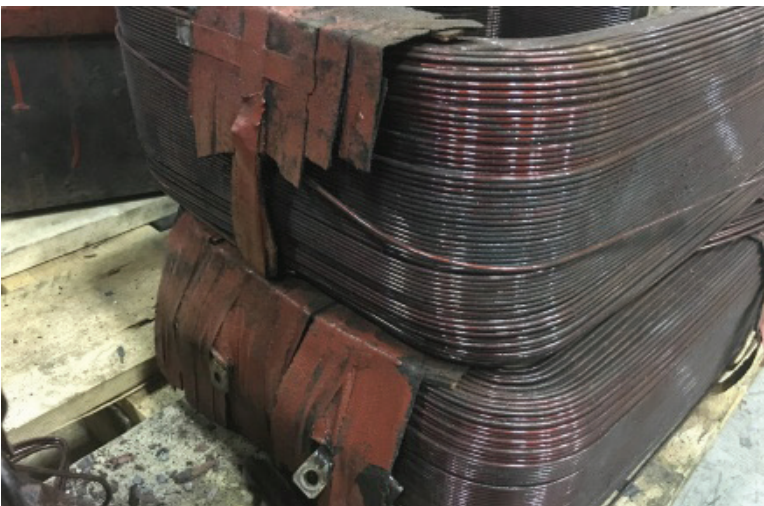
These field coils were still working and literally fell apart once touched.
