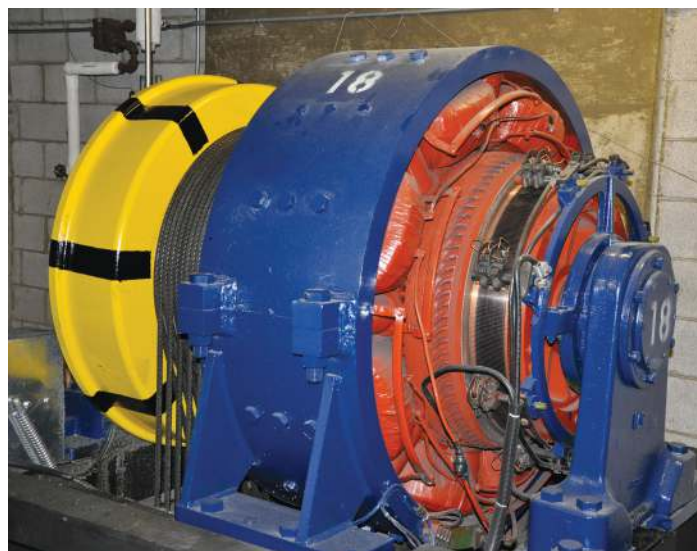
A gearless unit being serviced
