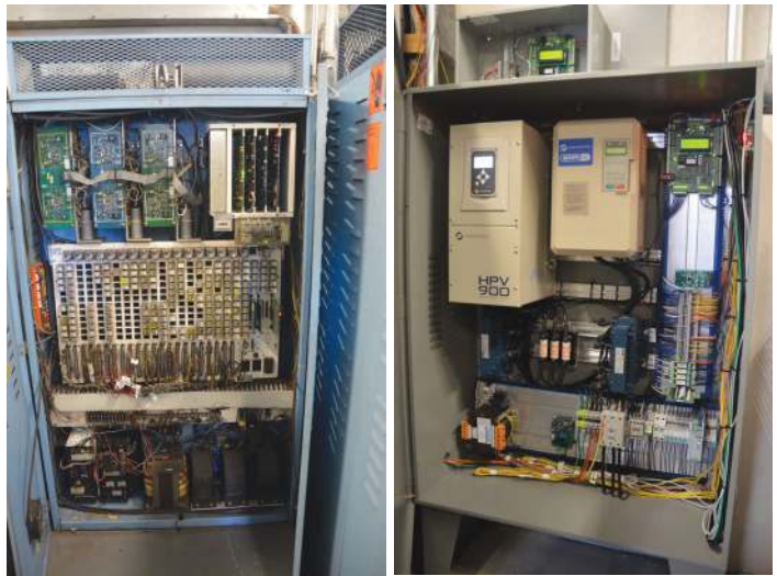
(l-r) A controller upgrade, from single-phase Otis MRVF equipment of 1980s vintage to an SRA (AC traction) machine with power-line regenerative kit from SmartRise Engineering, Inc. (photos by Capitol Elevator)
