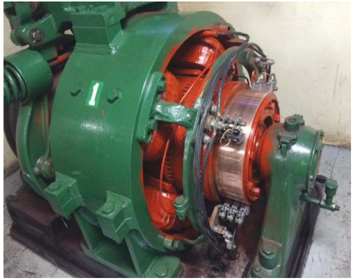
New insulation and reseat after a clean and undercut
