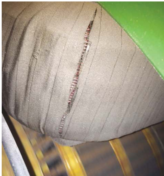
The cracks in this machine's coil insulation can easily be overlooked, as replacement costs thousands of U.S. dollars.
