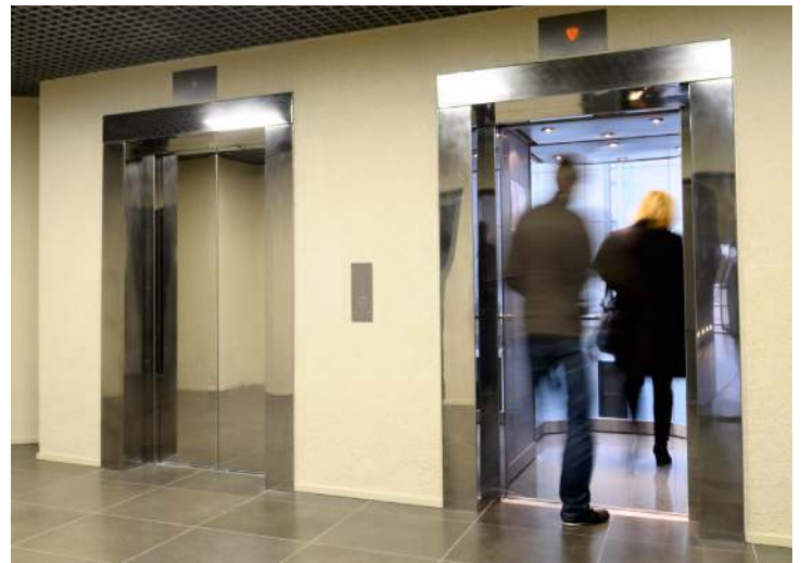
An elevator motor's standard life expectancy is about 25-30 years. Proper preventative maintenance depends largely on the working environment and usage of the equipment.
