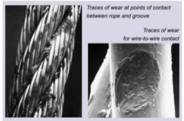
Example of rope damage
